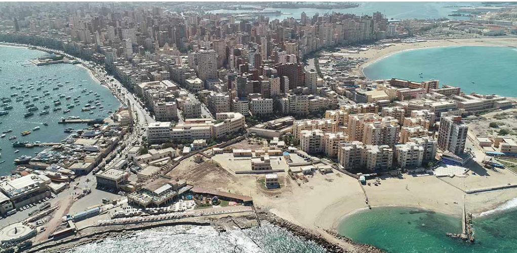
Picture 9: Alexandria-Abou Qir Metro Line Project
