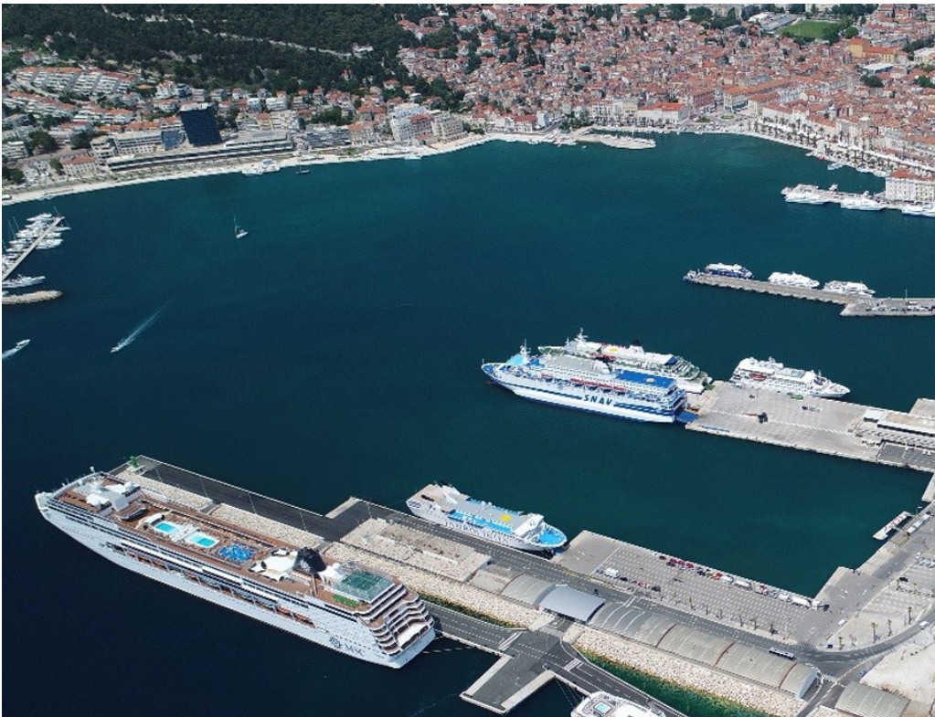
Picture 5: Exterior of the Split Port Breakwater
