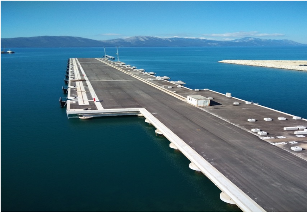
Picture 1: Example of a project financed with the assistance of the IBRD: Port of Ploče, Main Terminal
